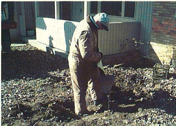
Abandoned water well being plugged by a licensed water well driller.
